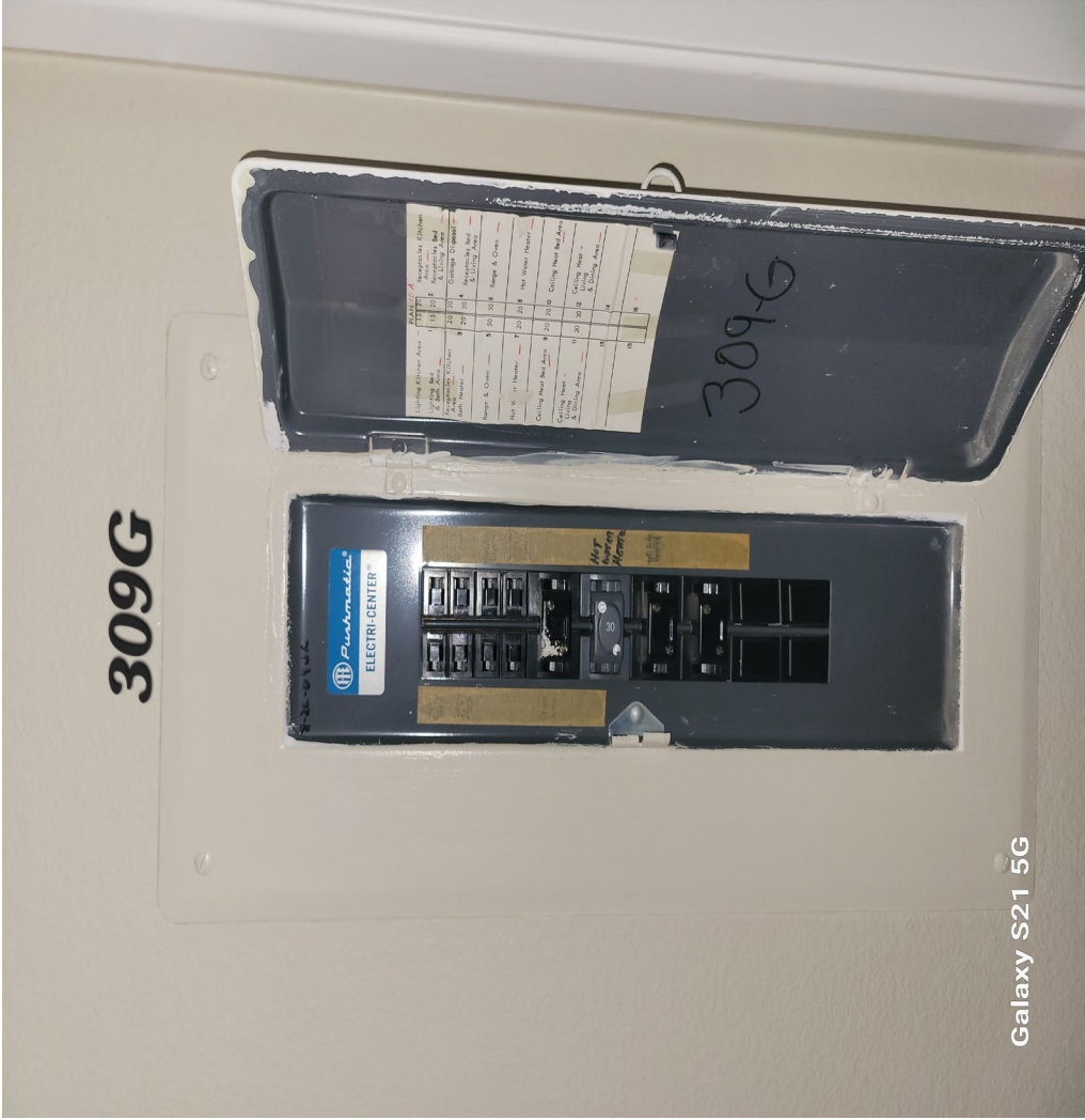
Existing Panel Before
