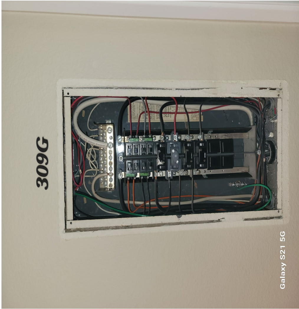
Before Panel Replacement
